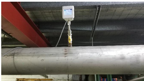
Display is facing the user. This makes it easy to read the flow rate
