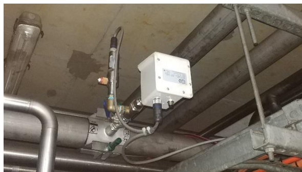
Display is facing the roof.
